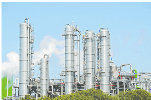
Figure 3 Distillation towers at a bioethanol plant.
